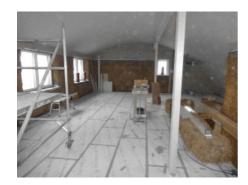
Currently under construction, Haven Cottage is a two-storey load-bearing straw bale house aiming for Passivhaus certification. It has a 'passive slab' foundation, floating on 400 mm of EPS. A timber barrel-vaulted roof filled with 450 mm of Warmcel and covered in standing seam aluminium. Hoping to rely on electricity, aided by a 4 kW solar PV installation.
