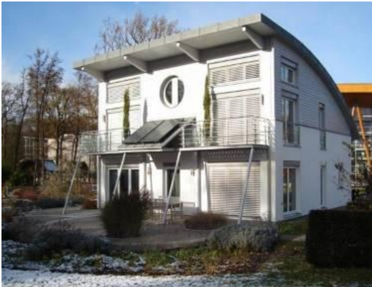
Weber pre-fabricated timber frame Passivhaus, Germany (photograph KP ArCreation)
